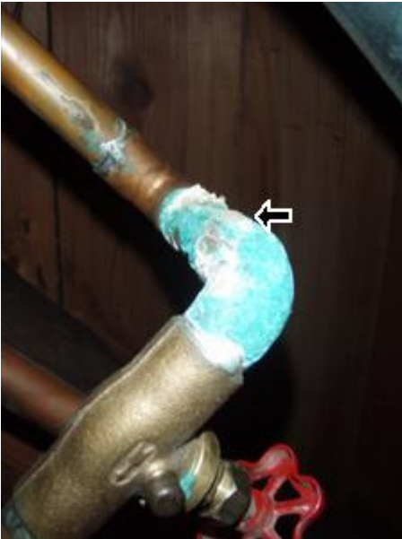
4.2 Picture 1 clean pipe
