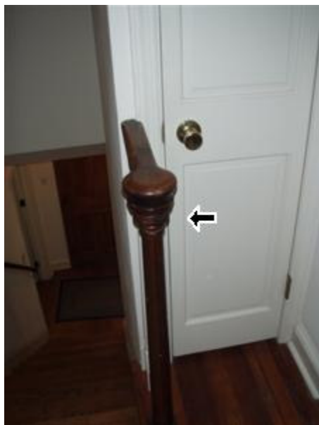
8.3 Picture 1 tighten rail
