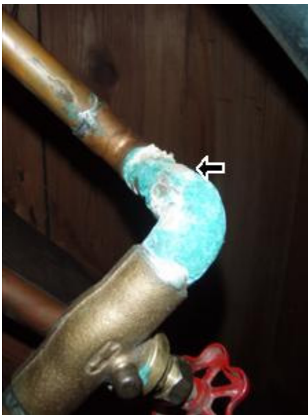
4.2 Picture 1 clean pipe
