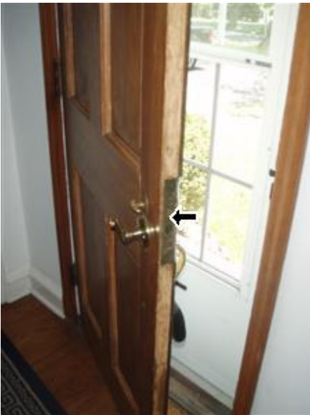
2.1 Picture 1 repair lock
