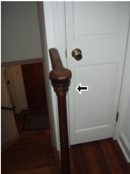
8.3 Picture 1 tighten rail
