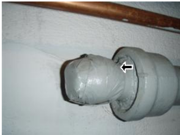
4.0 Picture 1 properly seal
