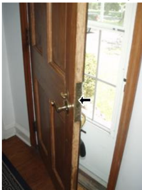
2.1 Picture 1 repair lock
